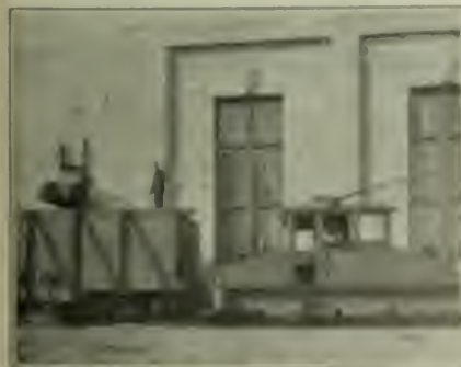
250-HORSEPOWER ELECTRIC LOCOMOTIVE AND COAL CAR
